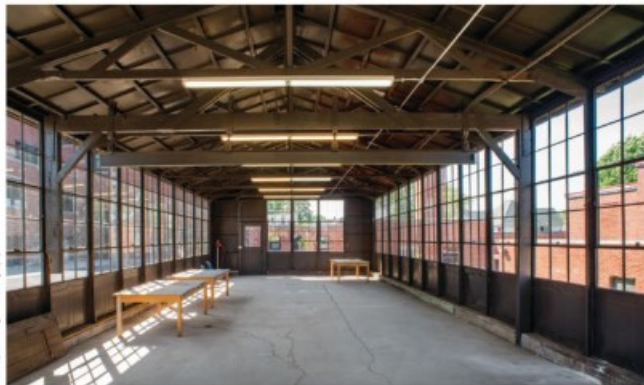
BACK TO ROOTS The property's original greenhouse had been converted to a field house for sports equipment. It has now been reimplemented as a greenhouse for residents' use.
